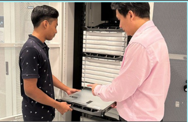
Data Centre Lab (Server management)
