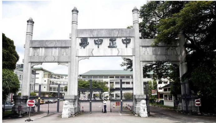
Chung Cheng High School (Main) 中正中学总校 Goodman Road near Dakota MRT. Built in 1968 as an education institution Gazetted for Preservation as a National Monument in 2014 Photo Credit: The Straits Times
