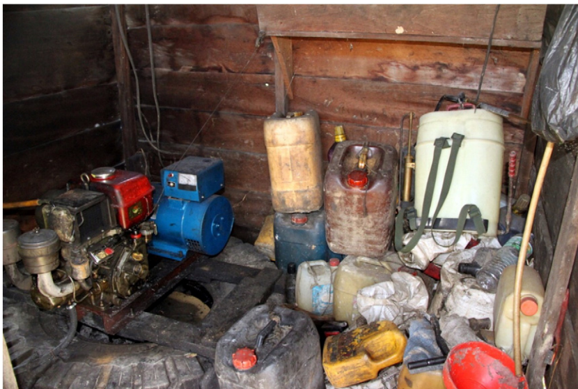
Fig. 9. A 15 kW diesel generator and discarded fuel cartons near Long Wat, Murum, Malaysia.
