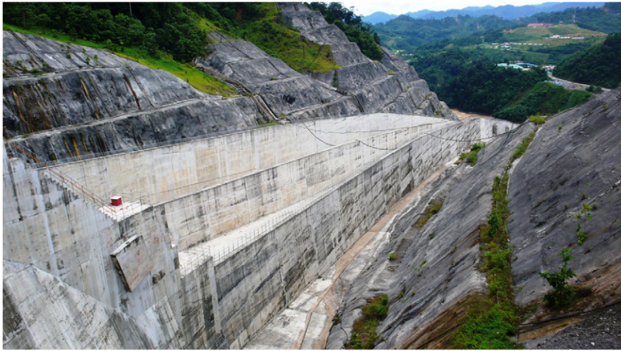
Fig. 3. The spillway of the Bakun Hydroelectric Project.
