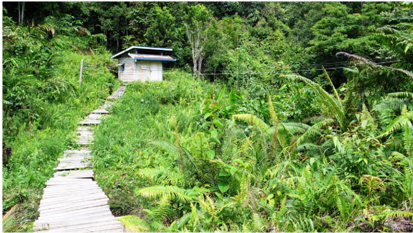
Fig. 5. The 10 kW micro-hydro unit at Long Lawen, Belaga, Sarawak.
