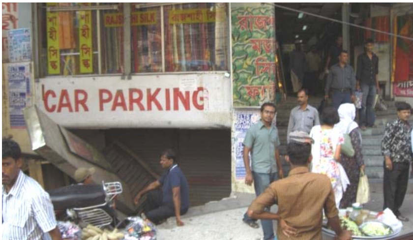
Figure 1: Basement in Dhaka presumably planned as parking space then used for shops which have now been demolished in enforcement action.
