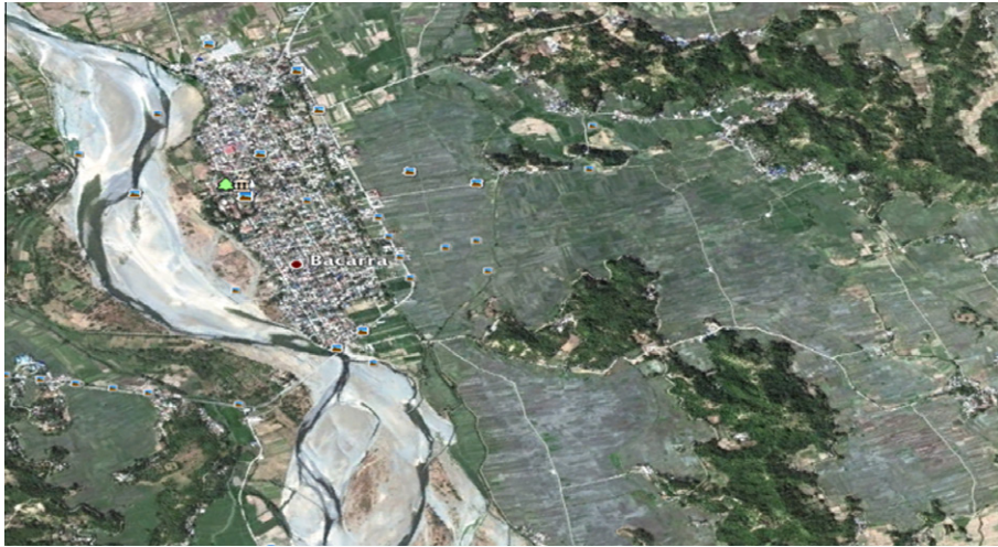
Fig. 3. Satellite photo of the zangjera farmlands traversed by the Bacarra-Vintar River. Note the densely populated town center, small farm holdings and the heavily silted, expansive river, which makes a permanent dam infeasible. Heavy siltation and a monsoon climate is the main source of persistent flooding in the zangjeras, requires a reliable method of mobilizing labor for constant repair. During periods of drought, the zangjeras need a fair system to allocate scarce water. The atar system of property rights evolved to solve these twin problems. Source: Google Earth.
