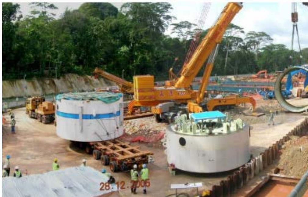
Fig. 5. Surface activity at a drilling site
