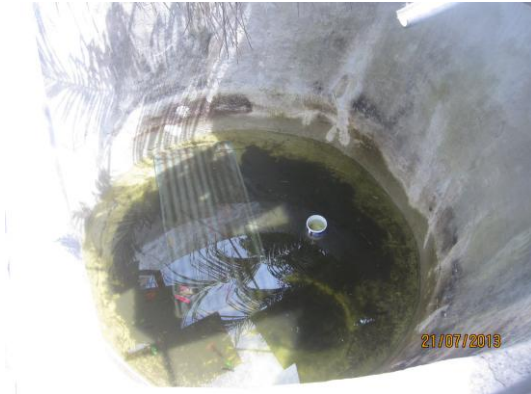
Pic15: Lack clean water is a major problem.
