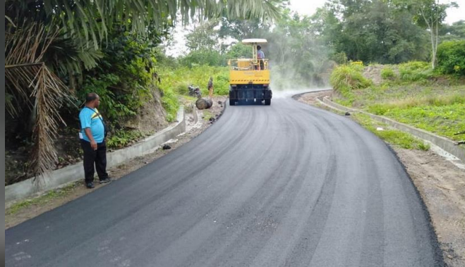
Infrastructure optimization by the government
