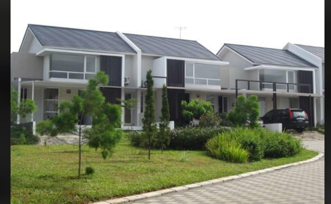
New housing residences, With total 34 housing today
