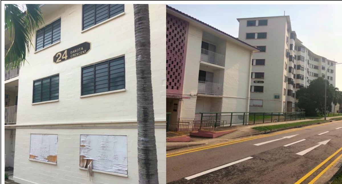
Low-rise blocks (3- and 7-storeys) at Dakota Crescent (Source: Author's own)
