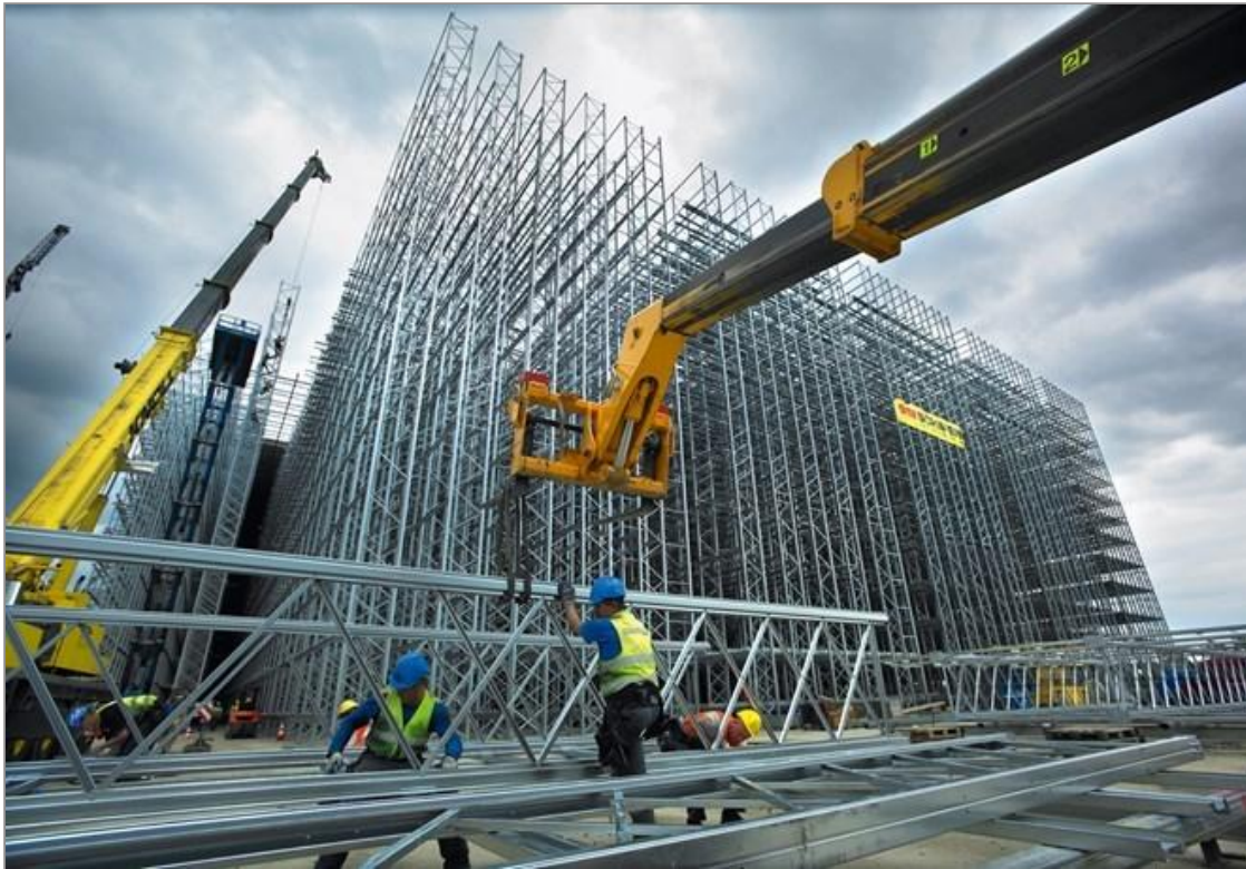
A construction site in Indonesia (Source: Financial Tribune)
